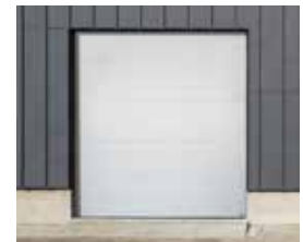
REPAIRED DOOR WITH AMARR 2747 REPLACEMENT SECTION
